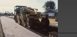
§Pulverize and blend full AC and predetermined portion of base/subgrade, cutting to required depth
