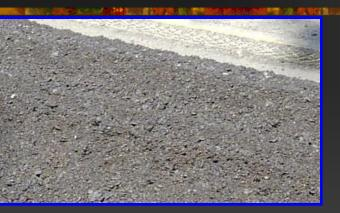
Chemical Stabilization •Portland Cement •Lime •Pozzolans (Fly Ash)
